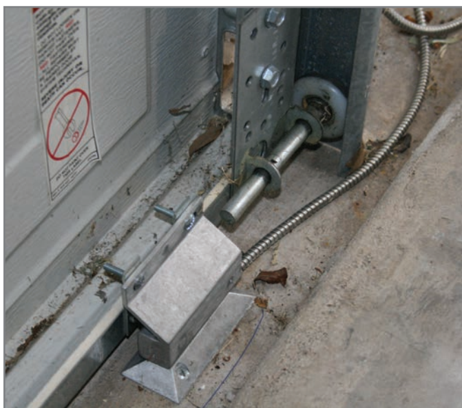
Photo 1 —These heavy-duty alarm contacts determine whether the garage doors are open or closed.
