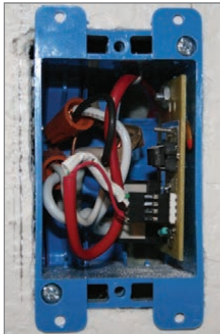
Photo 1 —Take a look at the final assembly. The board is mounted on the side, and two wires are pigtailed from the relay to wire nuts that control the AC power to the light. The four-conductor harness in red is the RS-485 line and 5-V power. This installation certainly won't endear me to any building code inspectors, but it works reliably.
